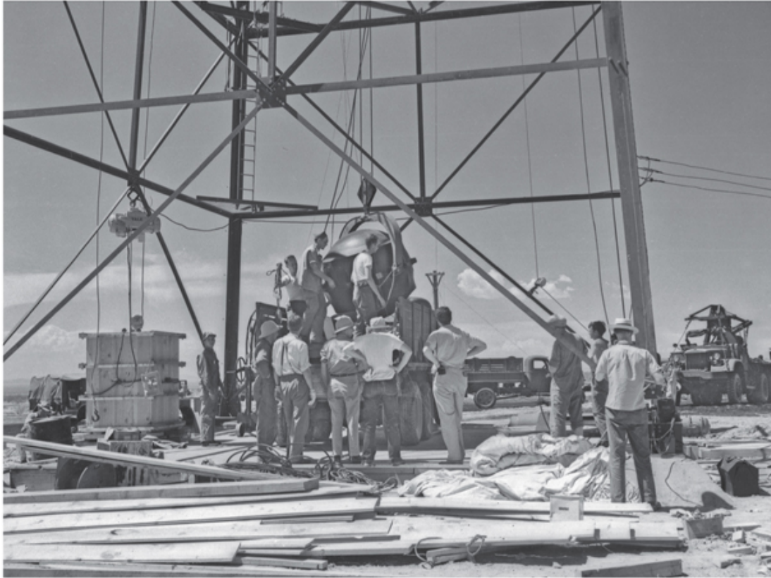
Unloading the Trinity bomb high-explosive assembly at the base of the 100-foot shot tower. Courtesy of Los Alamos National Laboratory.
