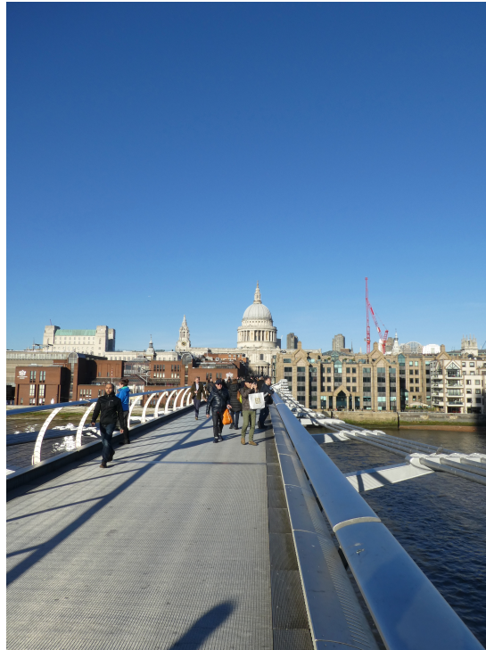
Figure 4.4.1 The Millennium Bridge
